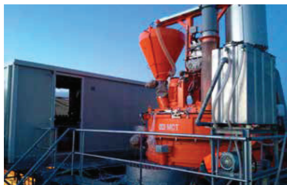
New mixing group during installation from the mixer platform
