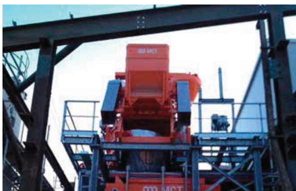
New mixing group during installation - Skip hoist side
