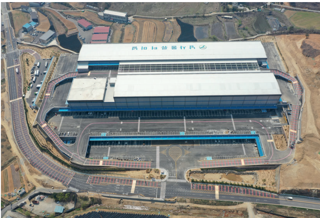
Namsa Cold Storage - first project of Jisan Engineering Co. Ltd
