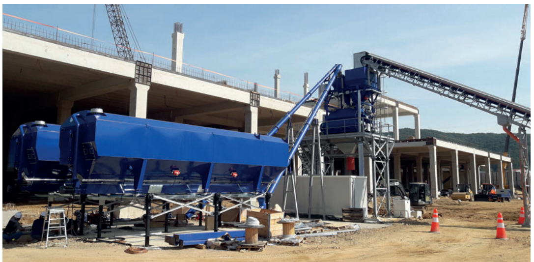
MCT Italy batch plant during installation
